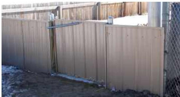
*Self-closing swing gate for pedestrians (springs on each side of gate). Metal culvert pipe at threshold blocks light.*
