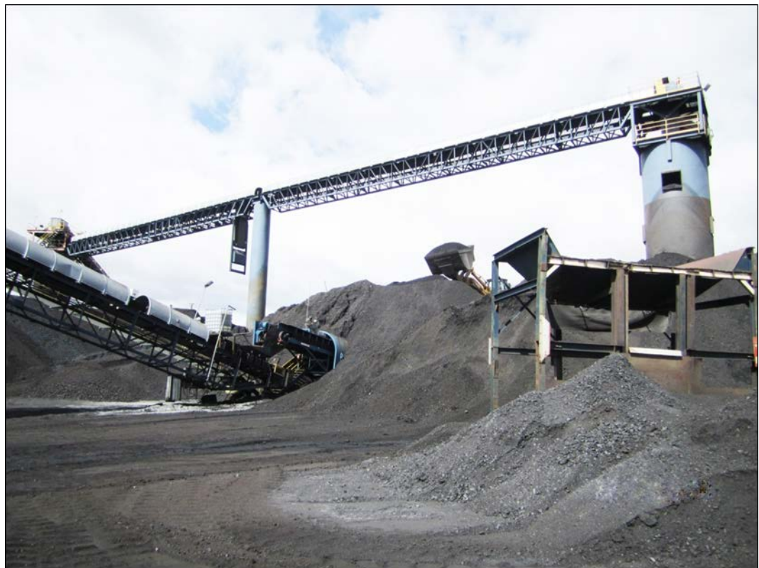
Figure 2. Load-out facility in Utah where coal from several mines is gathered and shipped to end users such as power plants. Source: Office of Inspector General.
