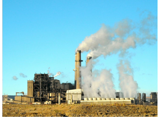
San Juan Generating Station in northwestern New Mexico.
