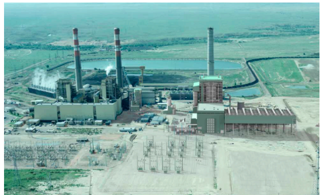
The Comanche power plant with a projected image of the number 3 boiler to the right. Photo by Xcel Energy.
